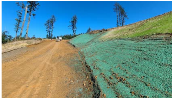
Hydroseeding a hillside
