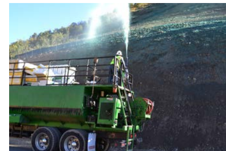
Hydromulch with Tackifier being applied
