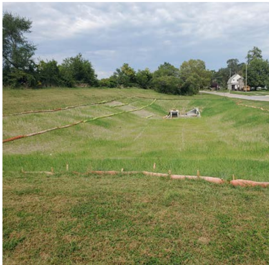
Wattles around a retention pond
