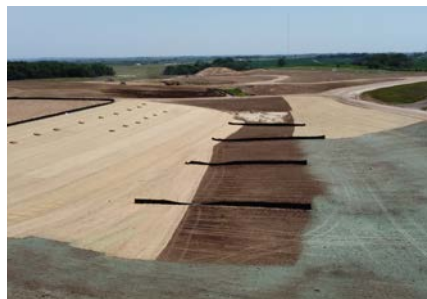
Silt Fence with Wooden Stakes
